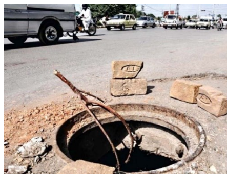
Figure .2: Opened Manhole
